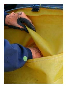
8. Should this not be the case deflate the liner slightly and adjust by pulling the liner through the access overlap flap at the far end of the liner.
